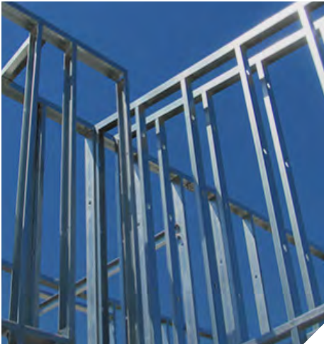
Steel Stud & Track (0.55 - 0.75 BMT)
