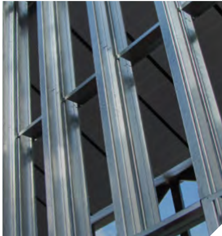
Structural Wall Framing (1.15 BMT)
